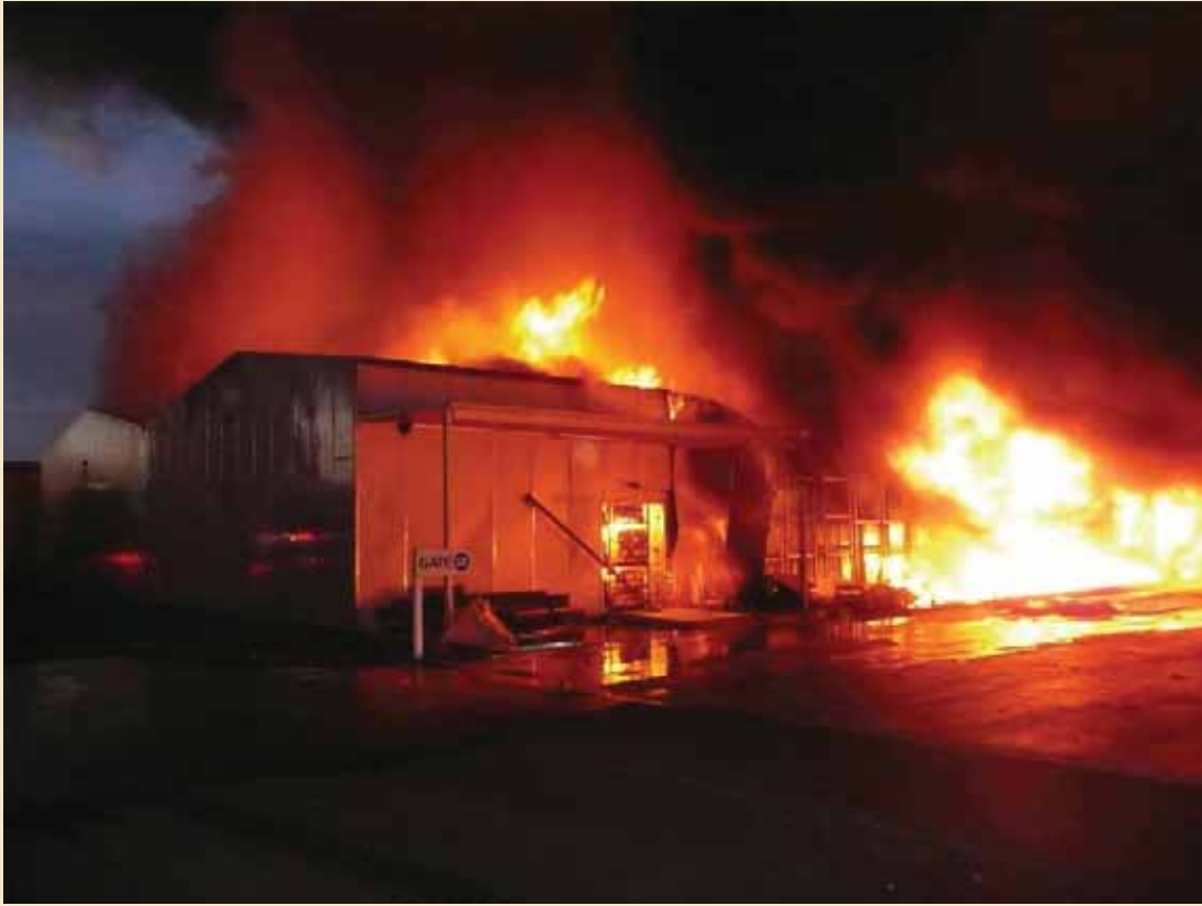
Figure 41: West Room involved in fire, 17:25
