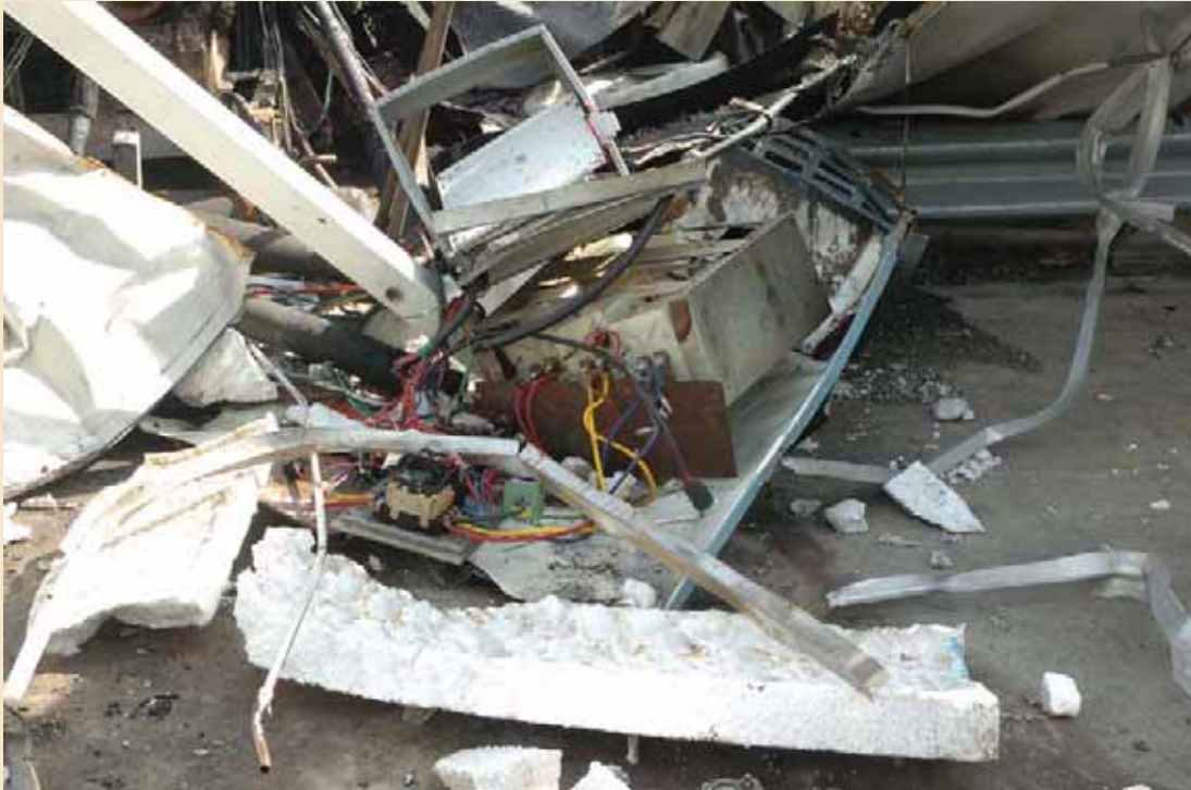
Figure 34: Electrical equipment from Plant Room 1 in location, close up
