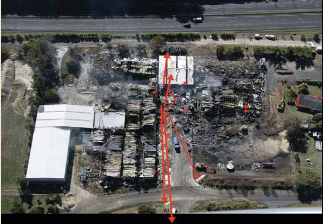
Figure 28: Aerial view of site showing calculated force vectors Plant room panels are lodged on the canopy.
