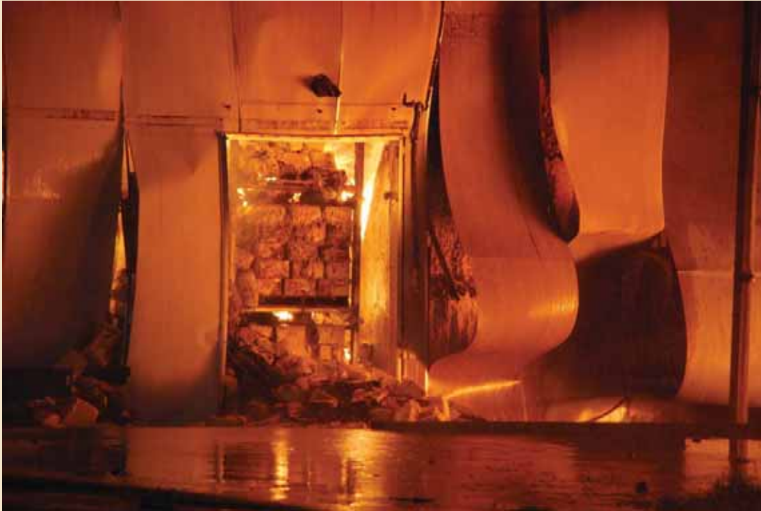
Figure 19: Delamination of wall panels of the West Room at about 19:45
